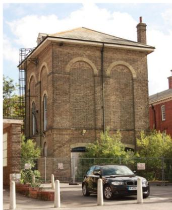
Directly to the west of the Cambridge Military Hospital within the courtyard of Gun Hill House is a tall yellow brick Water tower with wide eaves. The drawings for the Tower are dated November 1894 and the works signed off by Martin Wells in September the following year; the building is first seen on the 1897 Ordnance Survey Map. The plans were updated in 1905 and these
