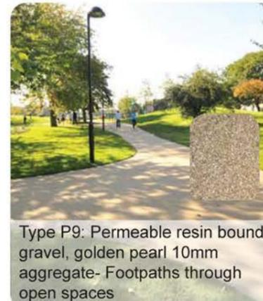
Type P9: Permeable resin bound gravel, golden pearl 10mm aggregate- Footpaths through open spaces
