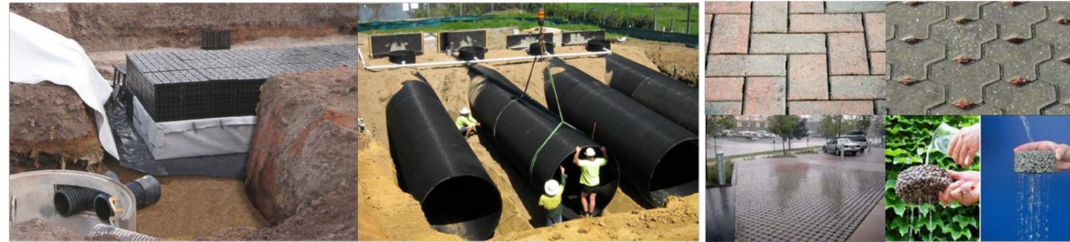
Phase 1 SUDS options - underground storage systems and permeable paving
