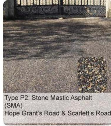
Type P2: Stone Mastic Asphalt (SMA)
