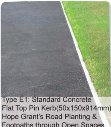
Type E1: Standard Concrete Flat Top Pin Kerb(50x150x914mm)
